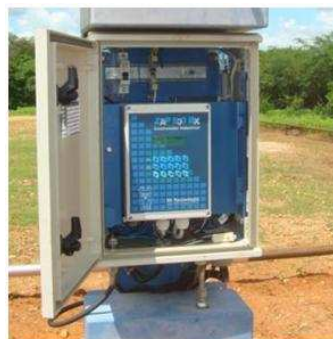
Figura 2.12: CLP usado no campo (Lorena - Mossoró/RN).
