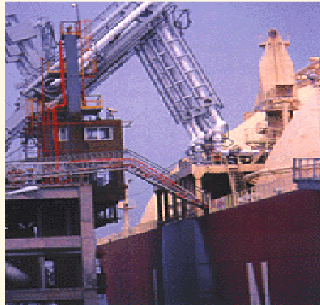
LNG receiving terminal, Chinese Petroleum Corporation, Yung-An, Taiwan
